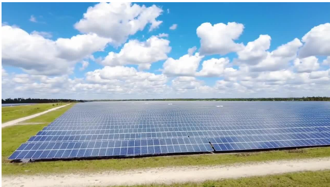
Figure 2: The large solar facility and battery storage system powers the Babcock Ranch community and surrounding region (Image credit Kaan Pala/WPTV)
