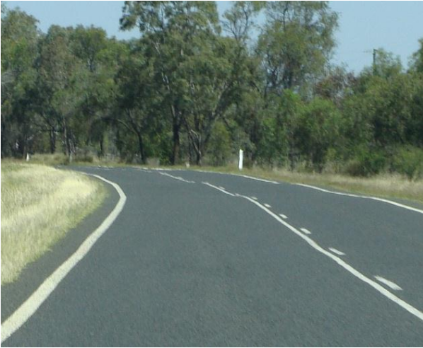
Some shoulder repair / widening works have taken place.
